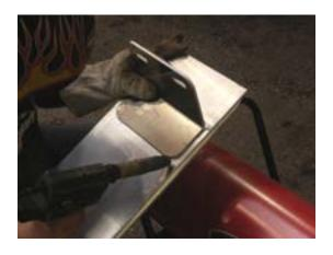
1C: Place bow legs flush on master bow at marks and weld in place (both sides).
