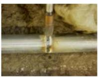
6A: Roll pipe and anchor pipe is supplied in 20' joints. Assemble and weld joints. Insert spline weldment in end of roll pipe and weld
